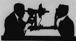
Measuring the Eye with the Ophthalmometer
