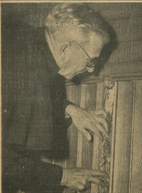
Considerable white ant damage has been discovered in S. Peter's Cathedral, Adelaide. The Chapter Vicar, Canon E. C. Loxa, is seen here inspecting some of the ravaged oak panels in the sanctuary.
