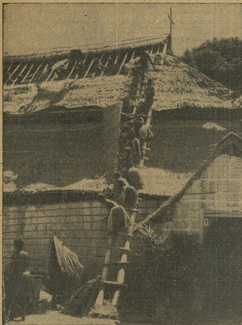
The winner of our snapshot competition this week is the Reverend N. E. G. Crutwell, of Menapi, New Guinea Mission, who sent us this picture of the roofing of a native church, S. Bartholomew's, Menapi, with sago leaf thatch. It is carried by girls and fixed in place by men. It costs nothing and lasts about ten years if well and truly laid.
