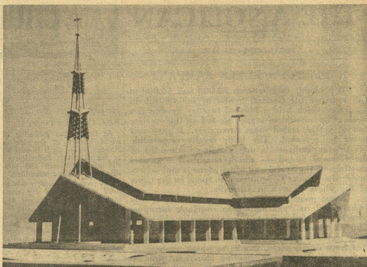
A model of the new Melanesian Cathedral of All Saints, Honiara, showing the roof built on two levels to assist the ventilation of the building.
