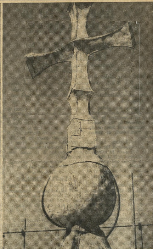
The cross on the dome of the historic S. Matthew's Church, Windsor, Diocese of Sydney. It is a facsimile of that on the dome of S. Paul's, London (but of much smaller size), and was erected in the 1840s. The wood has greatly deteriorated and the eight-feet cross encased in lead was considered to be dangerously insecure when the inspection was made on December 15 this year.
