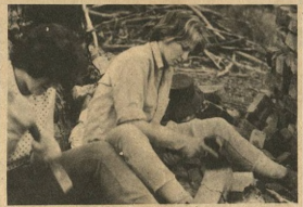
Sue Stewart and Julie Gibbes cleaning old mortar from second-hand bricks which were given to the camp.
